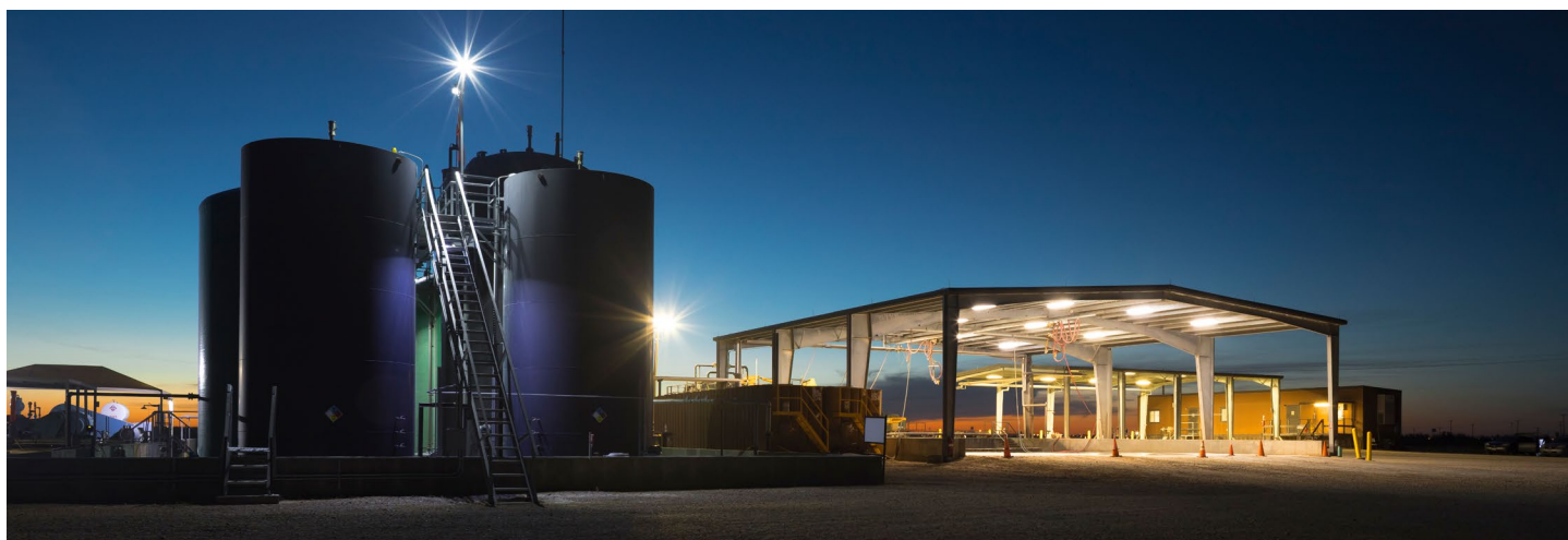
+ Slurry injection site in Pecos, Texas
