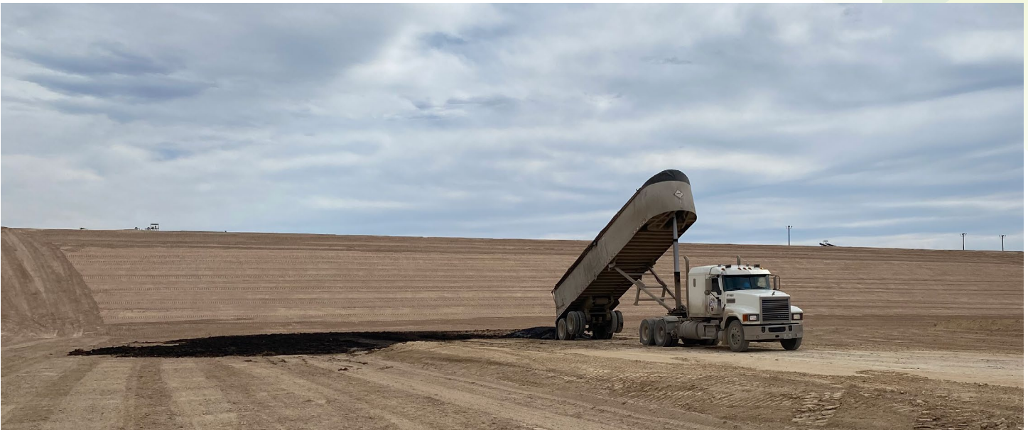
+ Leachate recovered is being blended into other solid waste and reinterred in our landfill.
